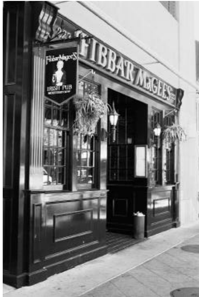
New storefront renovation on Castro Street. Entrances should be recessed from the facade, creating a small alcove.
