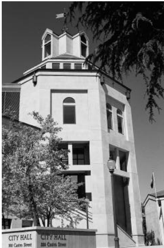
Mountain View City Hall
