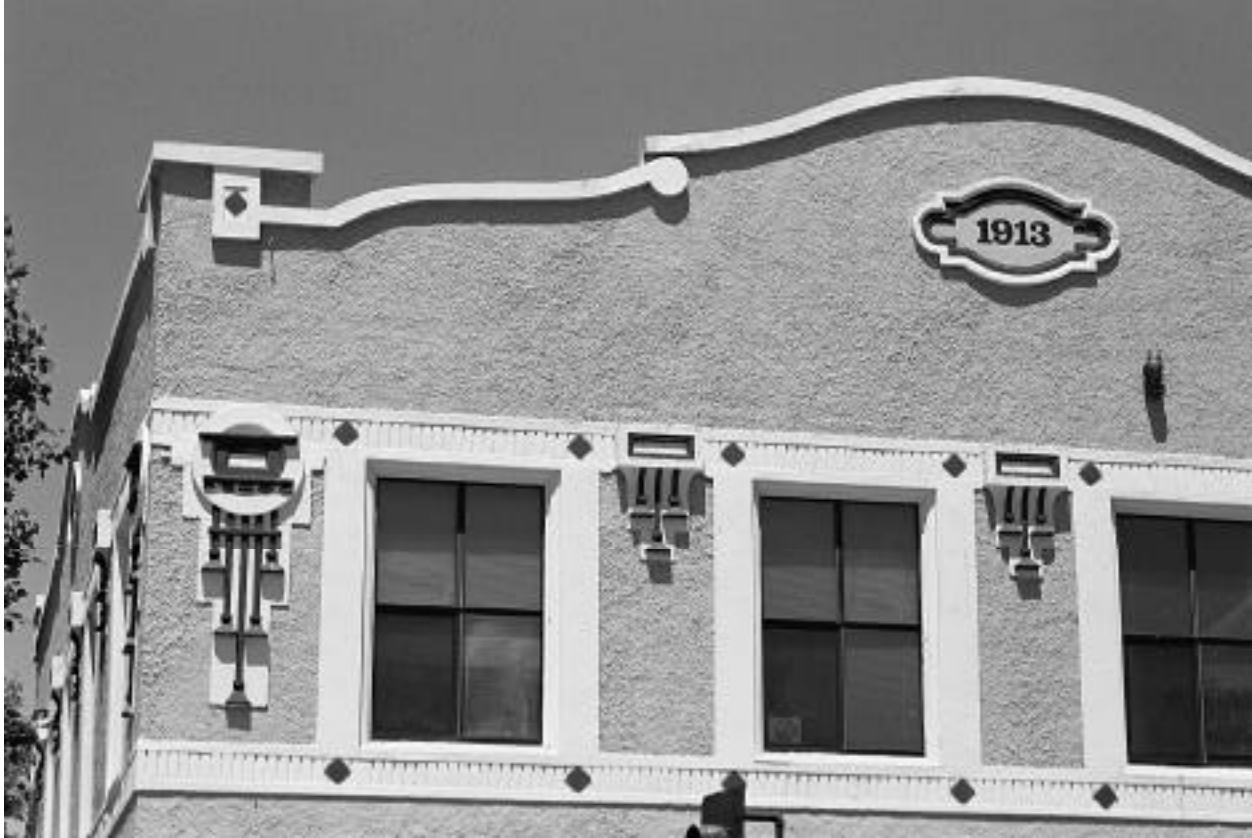
The Jurian Building, originally constructed in 1913.
